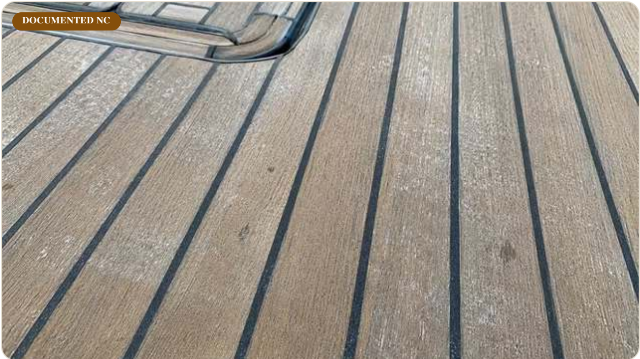
Close-up at 20 cm, reveals the blackening over 30% of the surface.
